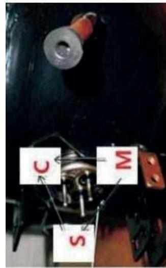
If the measure result is not in the range, it means the compressor has a problem. Change the compressor.
